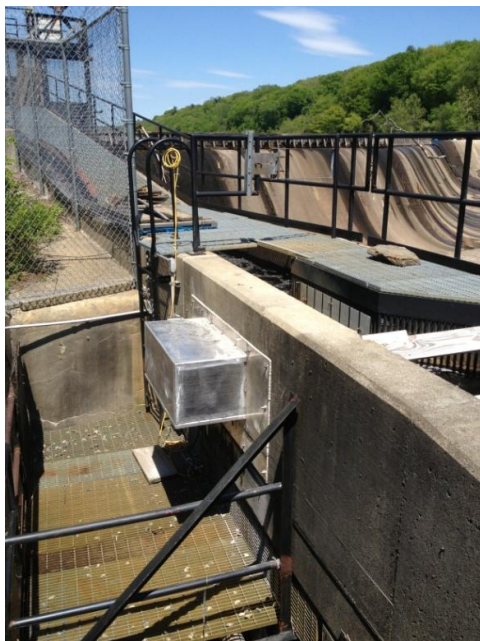
The old camera housing at Kinneytown fishway was wooden, dilapidated and unsecure. Tim Wildman designed a new one which was fabricated out of aluminum and Tim installed it with assistance from Anel- North America, the hydro operator. Note lack of spill over the dam.
